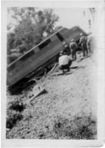
De-railed train near Jordan on the Minneapolis and St. Louis Railway.
